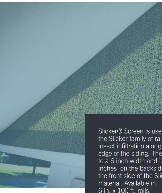
Slicker® Screen is used in conjunction with the Slicker family of rainscreens to prevent insect infiltration along the top and bottom edge of the siding. The material is precut to a 6 inch width and is installed with three inches on the backside and 3 inches on the front side of the Slicker rainscreen
