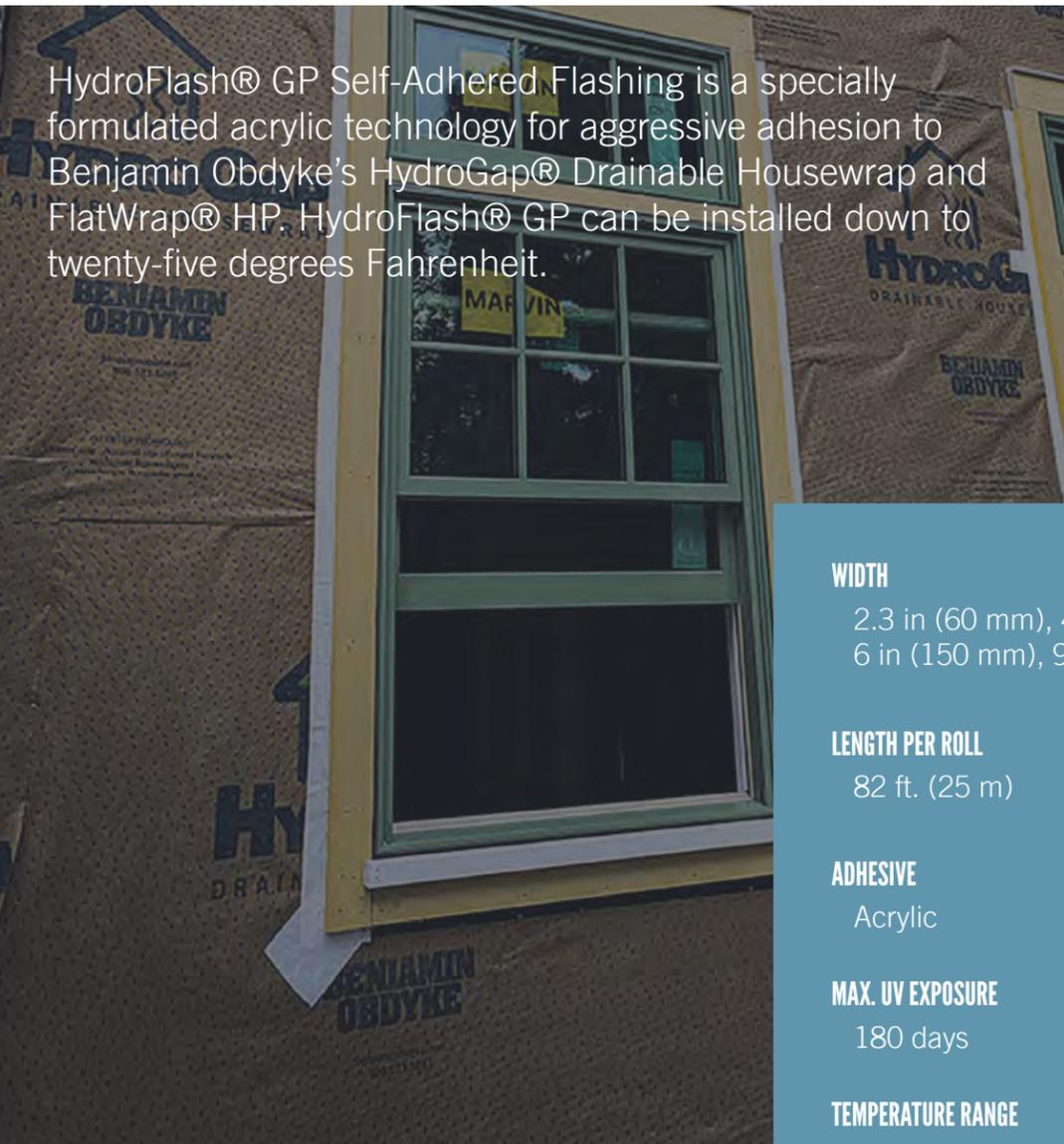
HydroFlash® GP Self-Adhered Flashing is a specially formulated acrylic technology for aggressive adhesion to Benjamin Obdyke's HydroGap® Drainable Housewrap and FlatWrap® HP. HydroFlash® GP can be installed down to twenty-five degrees Fahrenheit.
